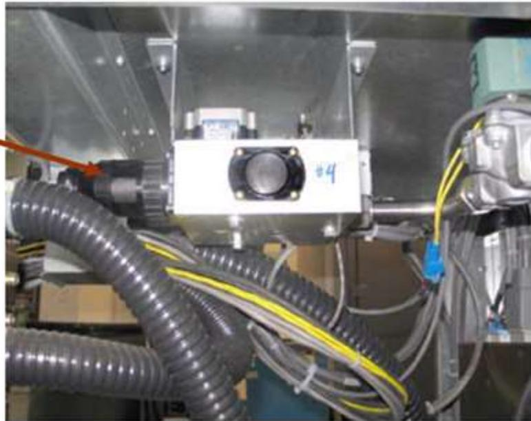
**Figure 2: UFCB Harness Location on Woodward Valve**
